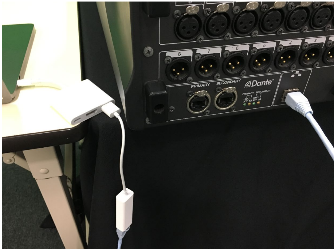
[Connect the console and Mac via LAN cable]
